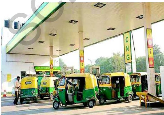
Fig - 3: CNG filling station
